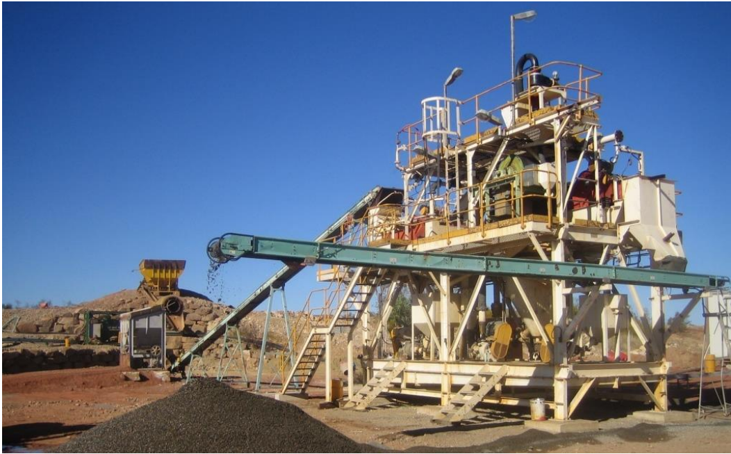
Processing plant at Merlin mine
